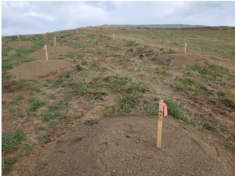
Photo 1 – Crown Excavating installed mounds of topsoil in the surveyed Phase 1 locations.
